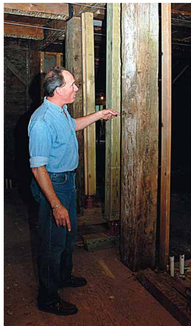
Examining an old, heavy beam donated by Jerry and Sally Law, Chris Guldner stands in one of the downstairs dining rooms. Beyond the beams are braces jacked up by Dan Schulte to straighten the 1802 inn.
